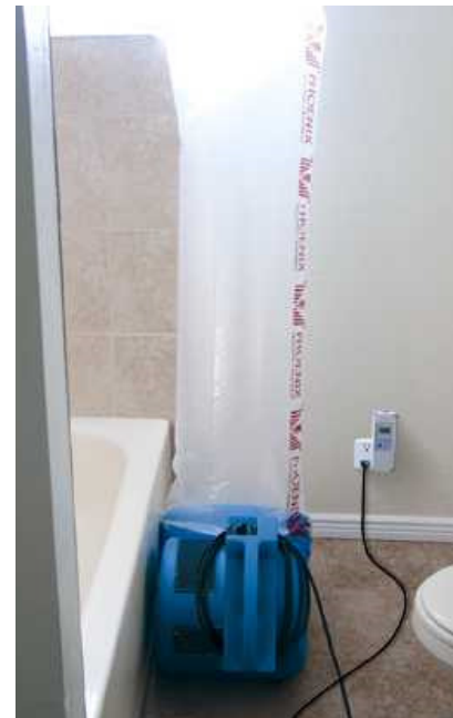
Air mover with ducting controlled by MB230 Exhaust Controller
